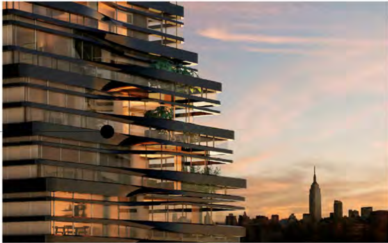
horizontal dark metal cladding
