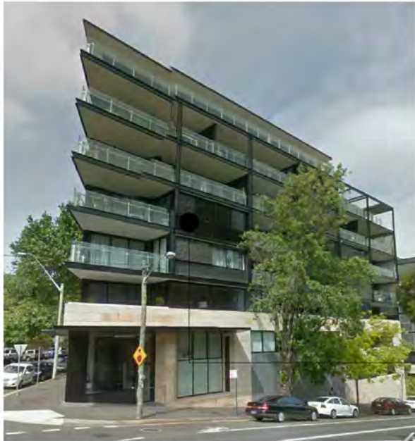
horizontal dark metal cladding
